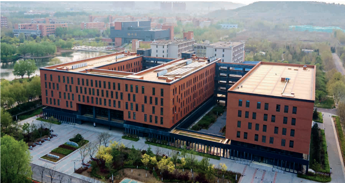
山东城市建设职业学院实验实训中心 Experimental and Training Center, Shandong Urban Construction Vocational College
