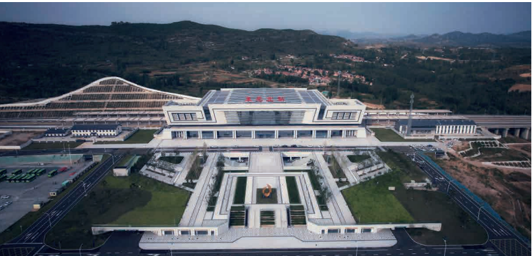
济莱高铁莱芜北站及其综合配套设计 Laiwu North Station and Integrated Ancillary Design of Jinan-Laiwu High-speed Railway
