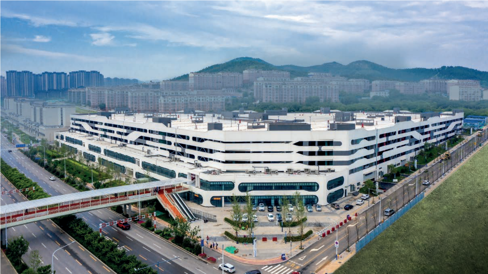
济南融创文旅城停车楼 Parking Building, Jinan SUNAC Resort
