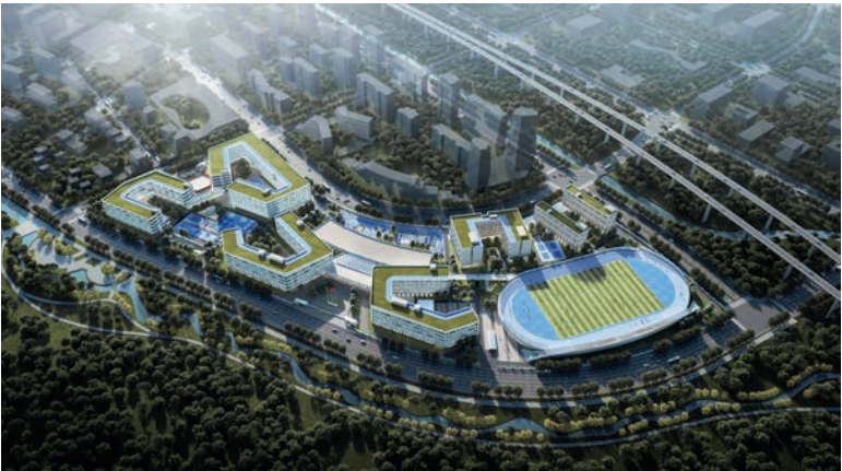
起步区都市阳台东组团国际学校 Start-up Zone Dushi Yangtai East Cluster International School
