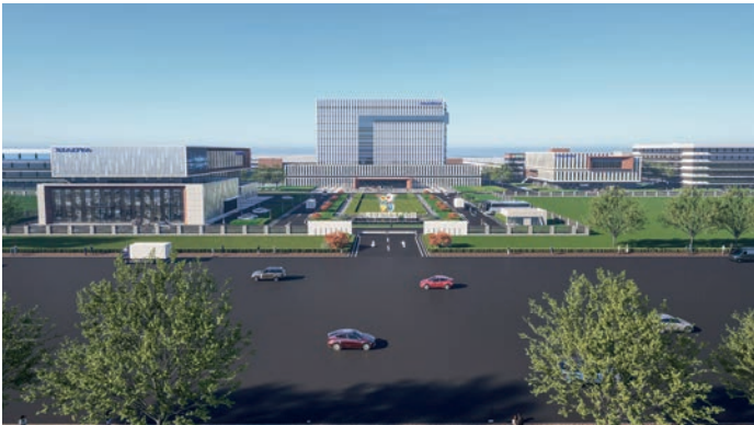
小鸭智能制造产业园 Xiaoya Intelligent Manufacturing Industrial Park
