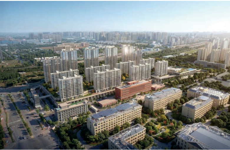
济南轨道交通2号线姜家庄停车场上盖保利公园上城 Poly Park Uptown above Jiangjiazhuang Depot of Jinan Rail Transit Line 2
