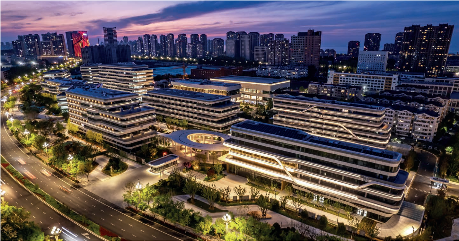
万华烟台工业园职工宿舍及配套设施 Staff Dormitory and Supporting Facilities, Wanhua Yantai Industrial Park
