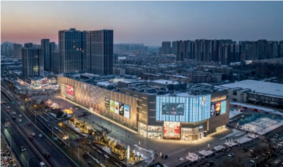
济南龙湖北宸天街 Longfor North Tianjie Street
