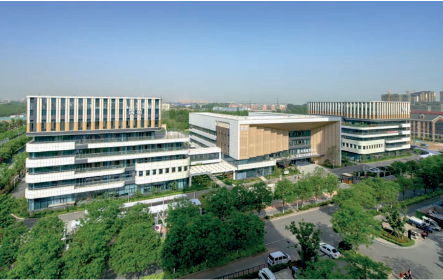
济南市历城区综合养老服务中心 Licheng District Comprehensive Elderly Care Service Center, Jinan
