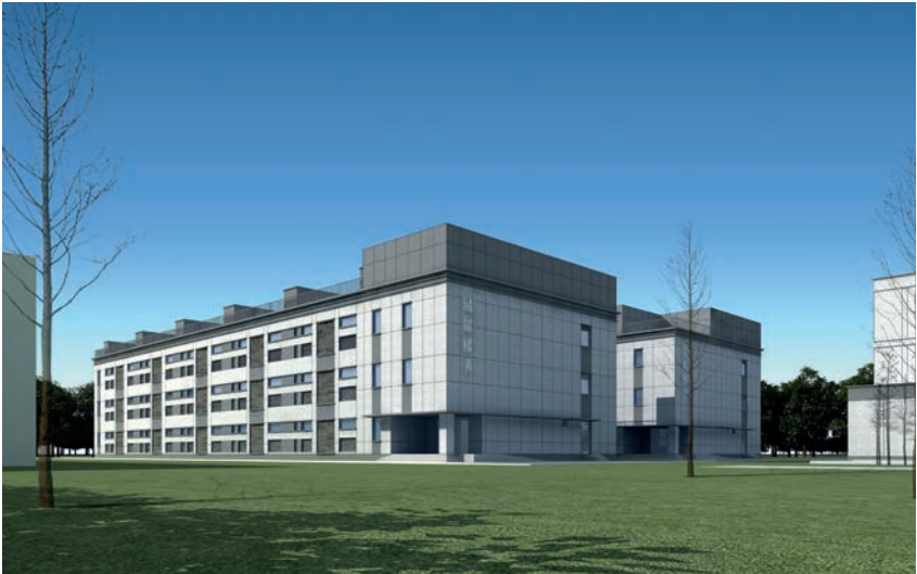
山东海琮200MW/400MWh共享储能电站 Shandong Haicong 200MW/400MWh Shared Energy Storage Power Station
