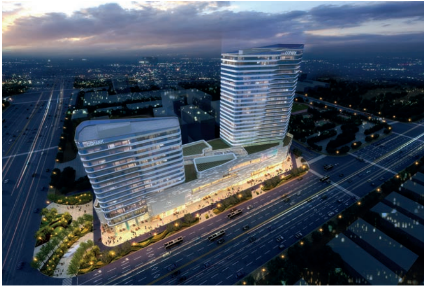
济南轨道交通2号线腊山地铁站上盖物业开发 Jinan Rail Transit Line 2 Lashan Metro Station TOD Project
