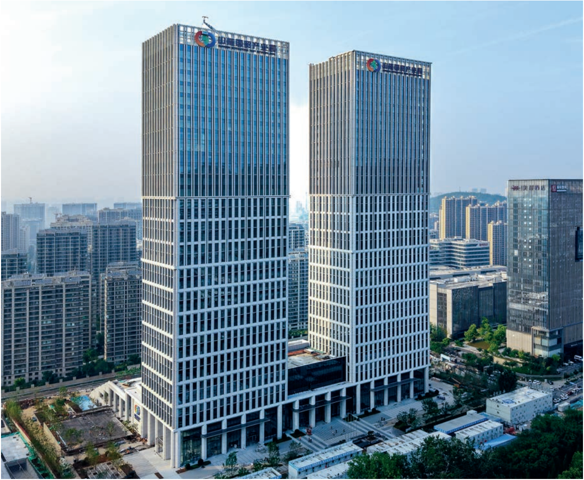
山东能源集团济南国际贸易产业园 Jinan International Trade Industrial Park of Shandong Energy Group
